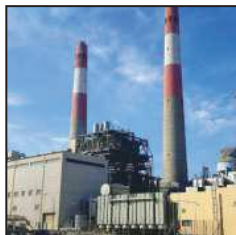
Lalpir Power Plant MuzzafarGarh
